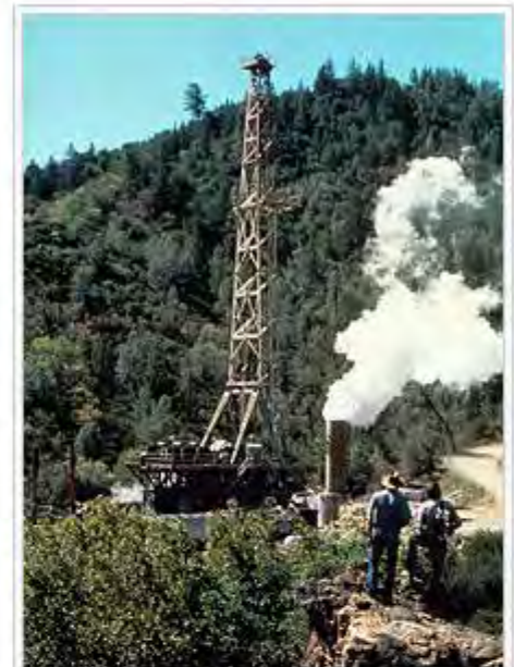
Drilling a geothermal well, 1977 □ (USGS)
