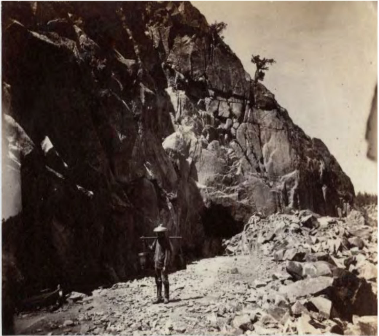
Hart 204. Heading of East Portal. Tunnel No. 8, from Donner Lake Railroad, Western Summit. This is not a Summit Tunnel, Tunnel No. 6, photo but it's interesting because it shows a Chinese worker probably carrying hot tea in the buckets for the other Chinese workers. The Chinese stayed much healthier than the Europeans who drank the frequently polluted stream water.
