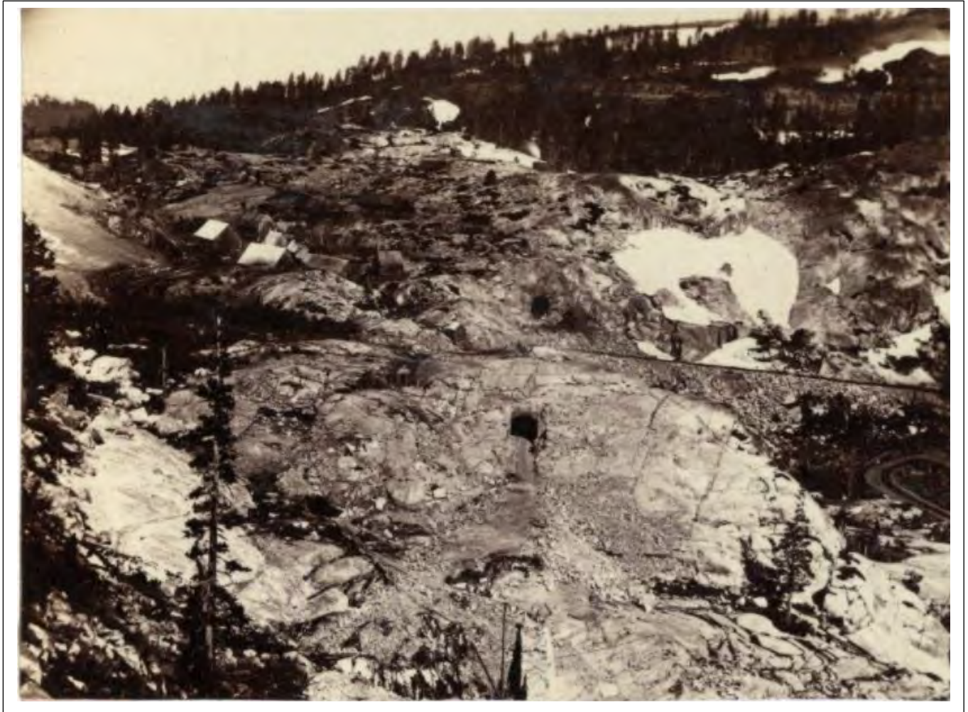
Hart 202. East Portals of Tunnels No. 6 and 7, from Tunnel No. 8. Looking west towards summit. Note buildings for housing the workers on the left, and the Dutch Flat and Donner Lake Wagon Road sloping down to the right from the Summit Tunnel east portal.
