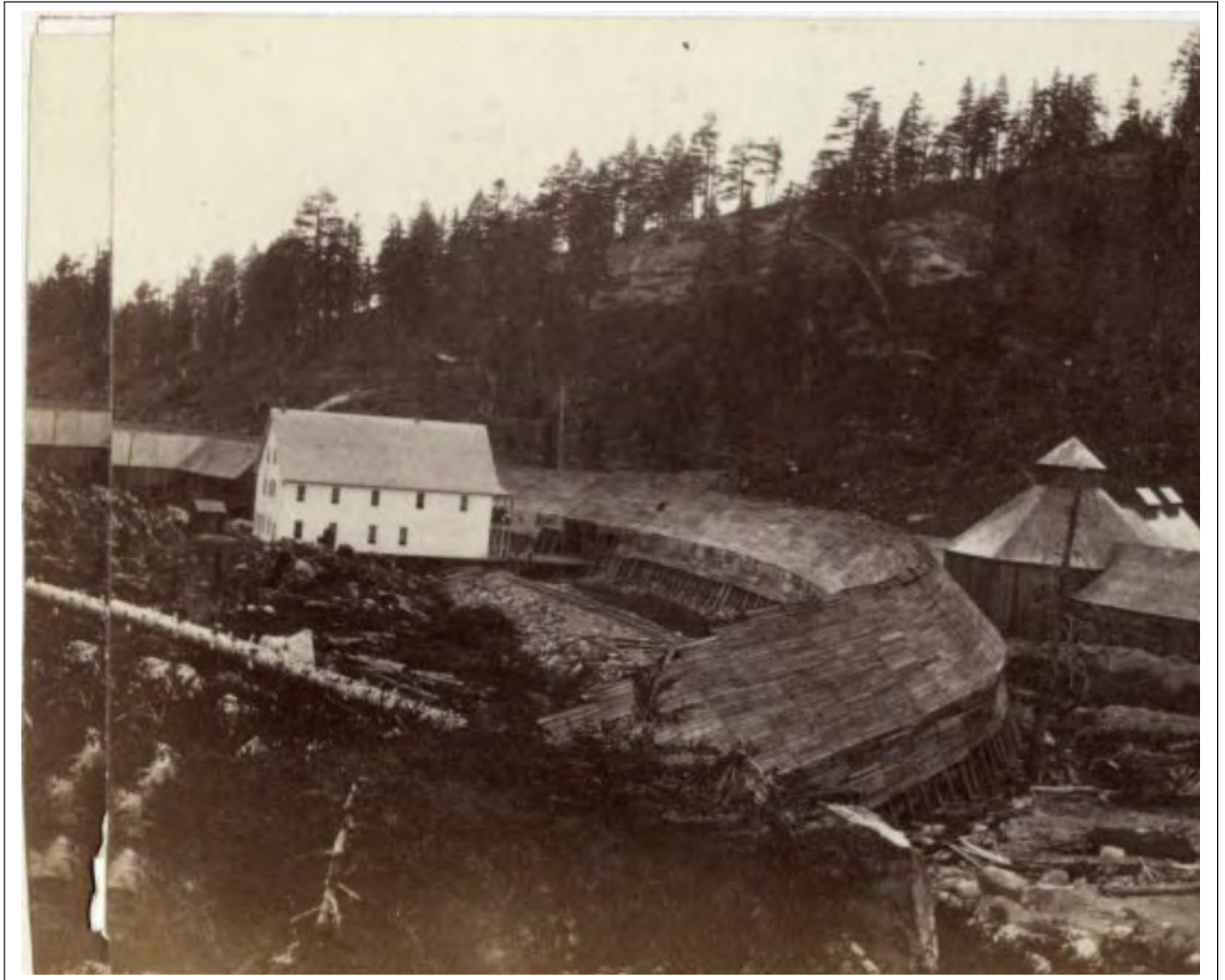
Hart 193. Summit Station. Western Summit. The snow shed closest to the viewer connects to the west portal of the Summit Tunnel almost below the photographer. Summit Hotel on left and turntable for turning helper locomotives on the right.
