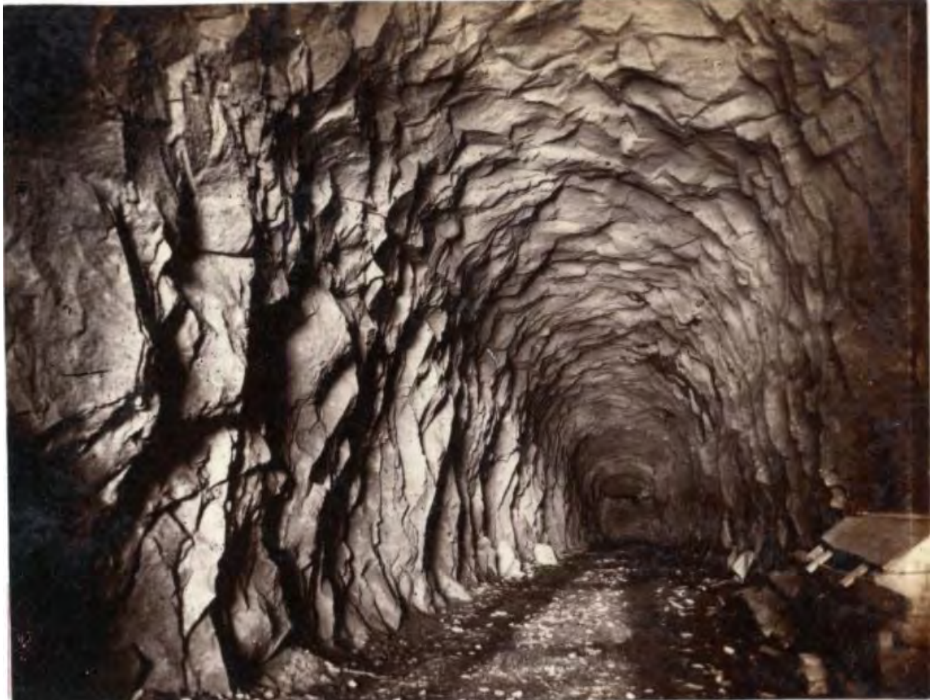
Hart 197. Summit Tunnel, before completion-Western Summit-Altitude 7,042 feet. The 7,042 elevation tells us that it is taken from the western portal with the setting sun lighting the tunnel. The eastern portal was at about 7,012 feet elevation, using the elevations from Gilliss' 1870 paper. Note the end of the tunnel where the arched "headings" are advanced ahead of the rectangular "bottoms."
