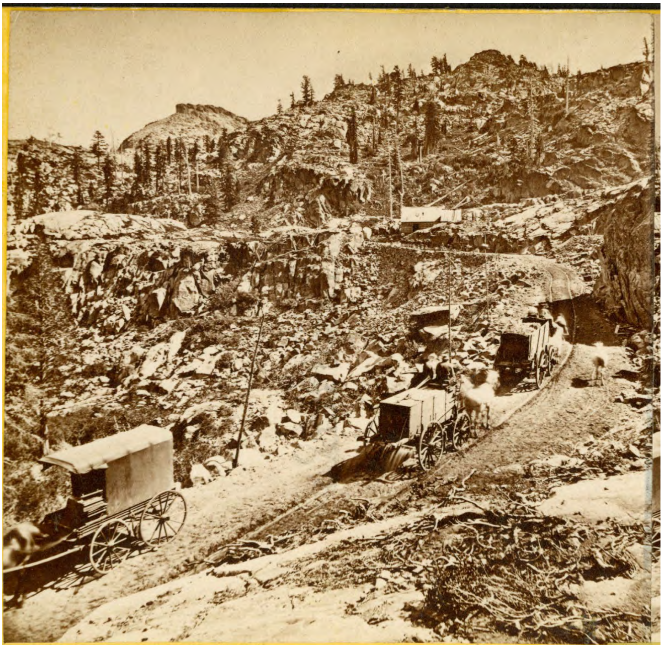
Hart 120. Wagons on Dutch Flat & Donner Lake Wagon Road. Alfred Hart's photography wagon lower left. Water wagon for dust control going uphill. Building in background is at east portal of Summit Tunnel.
