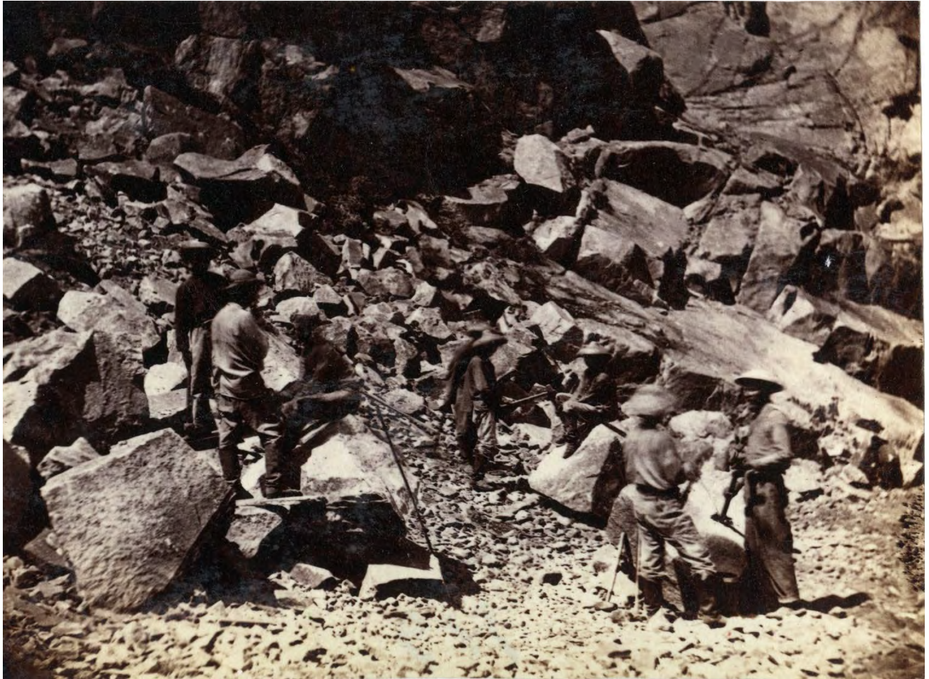
Hart 119. Chinese at east portal of Summit Tunnel. They are drilling holes in large boulders to blast into smaller pieces.
