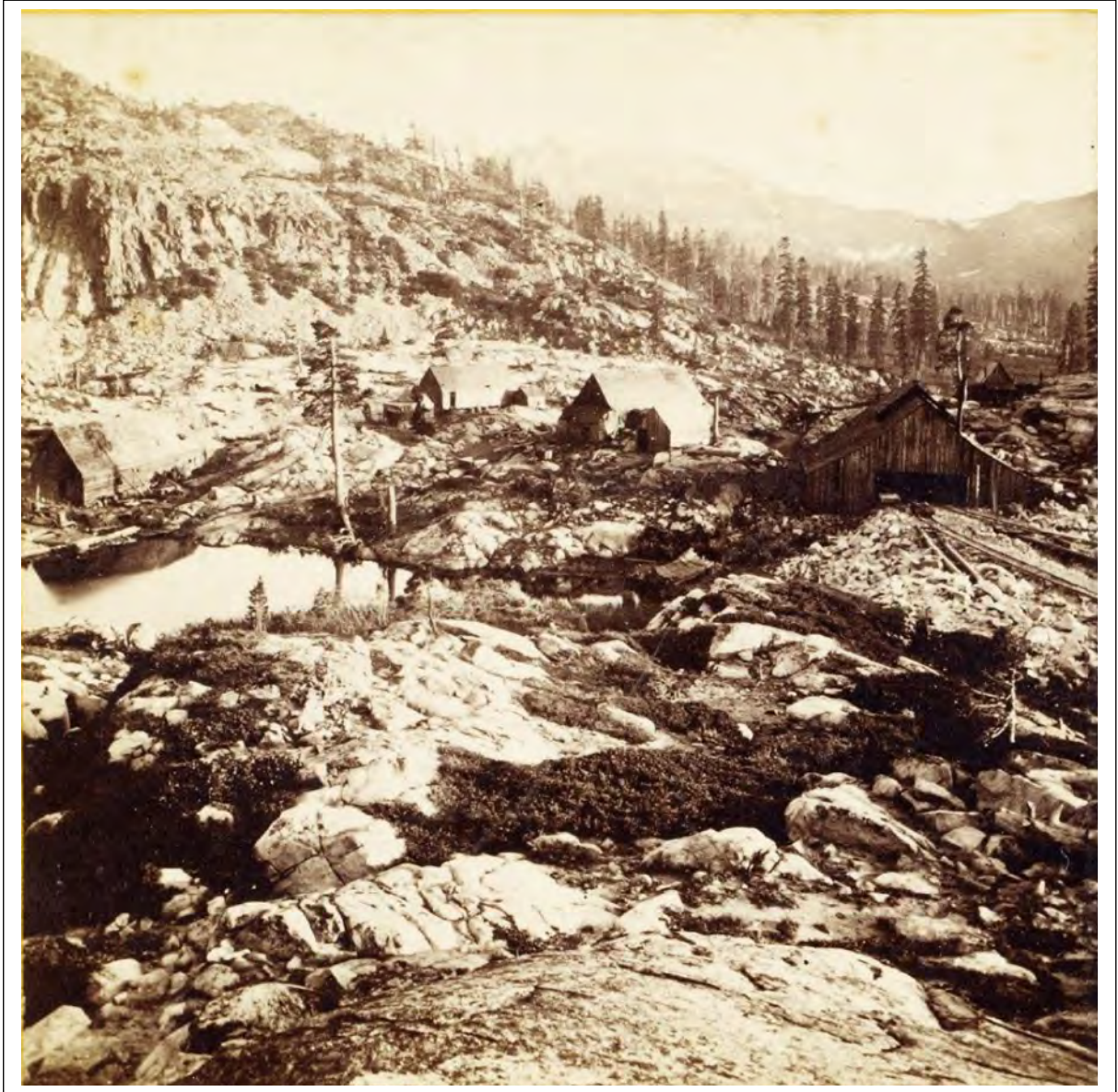
Hart 196. Shaft House over Summit Tunnel. American Peak in distance. The dark barn-like building is the shaft house which was constructed over the central shaft for the tunnel. An old steam locomotive boiler was used to power a hoist. Tracks for conveying the spoils from the shaft house to a dump site are on the right. Other buildings of the Summit Camp are in the background.
