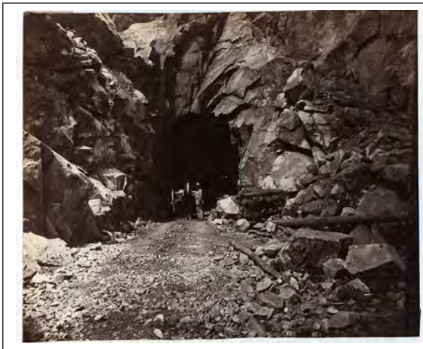
Alfred Hart #198. "East Portal of Summit Tunnel, Western Summit. Length 1,660 feet."
