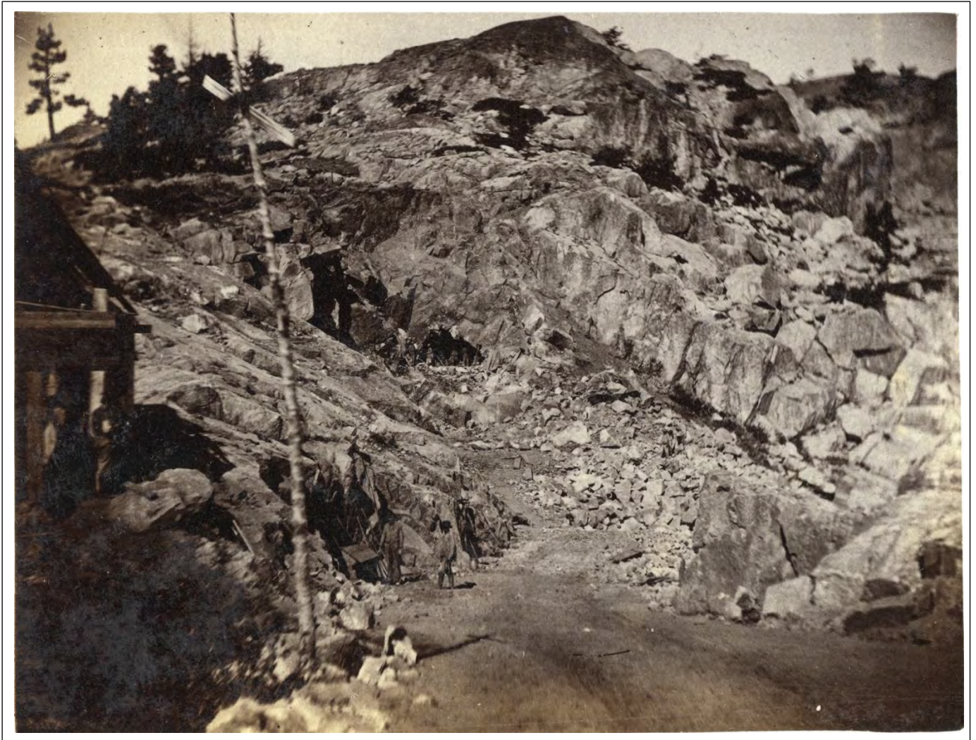
Hart 118. Summit Tunnel, Eastern Portal. Length 1660 feet on Western Summit.
