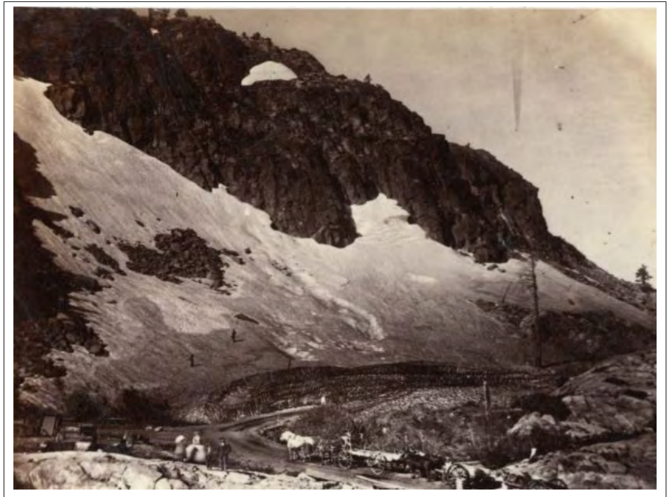
Hart 200. Bluff and Snow Bank in Donner Pass, Western Summit. Altitude 7,092 feet. The photo is looking west towards the top of the pass. Hart's elevation of 7,092 feet puts the Pass about 50 feet above the bottom of the tunnel at the west portal. The Dutch Flat and Donner Lake Wagon Road curves up towards the Pass. Note children at lower left with what looks like a snowman.
