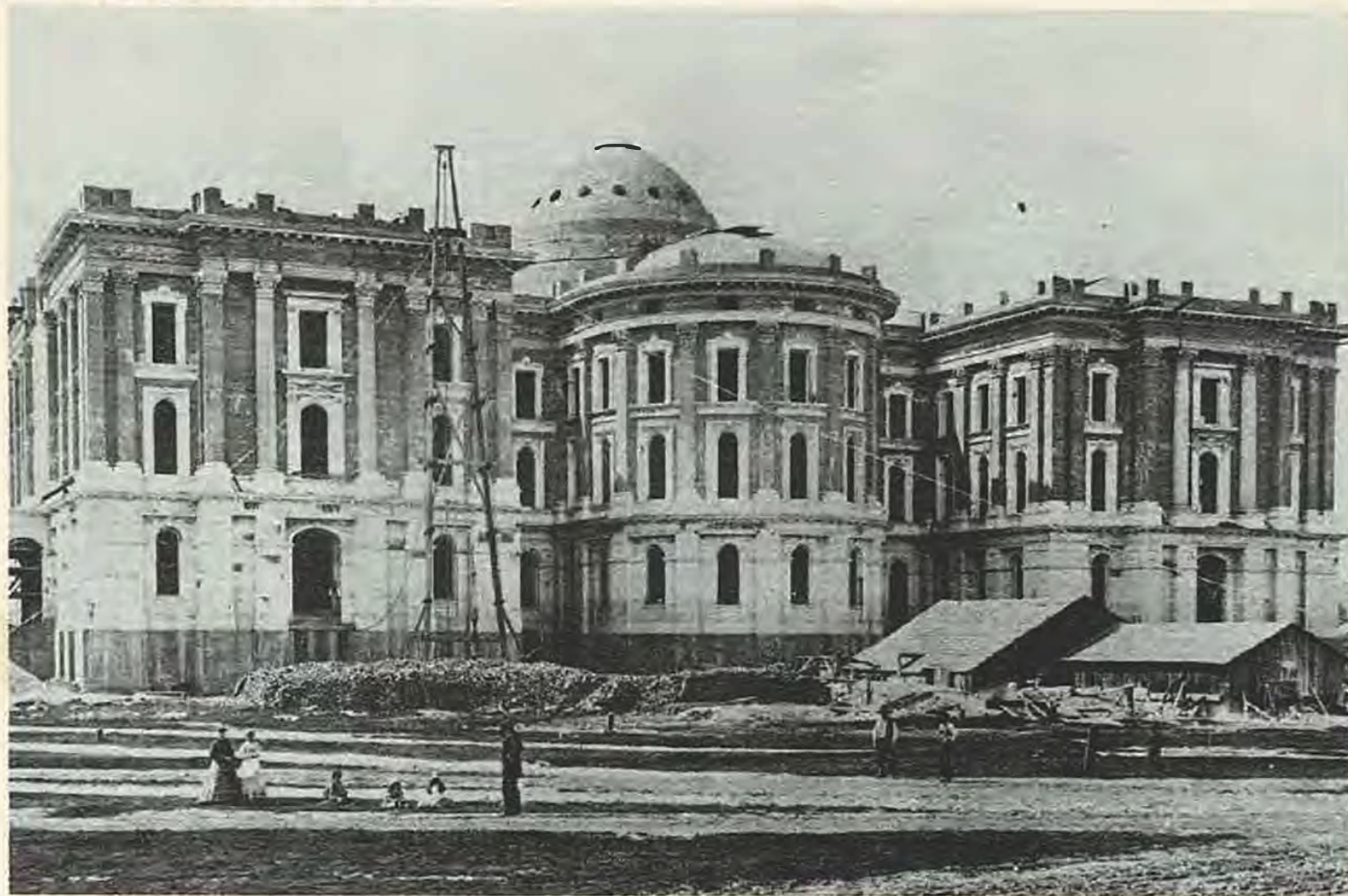
California's capitol under construction.
