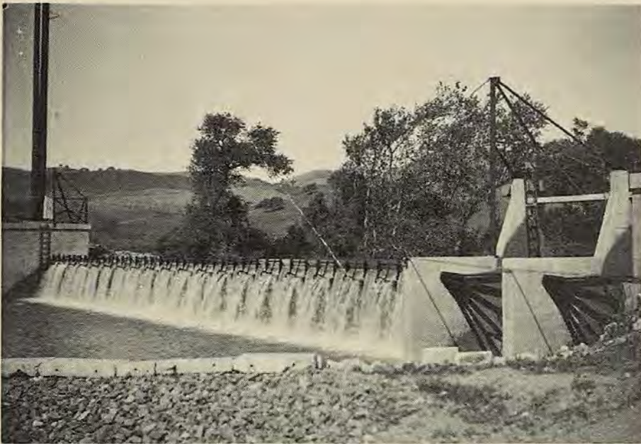
Coyote Percolation Dam. The cable car at right trips each dam section during excessive flows.
