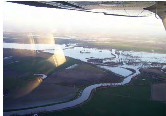
Figure 6, Fremont Weir (Sutter Bypass on left, and Yolo Bypass on right)
