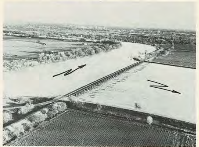
The Sacramento Weir during the 1950 flood. Flow directions in both the river and bypass are shown.
