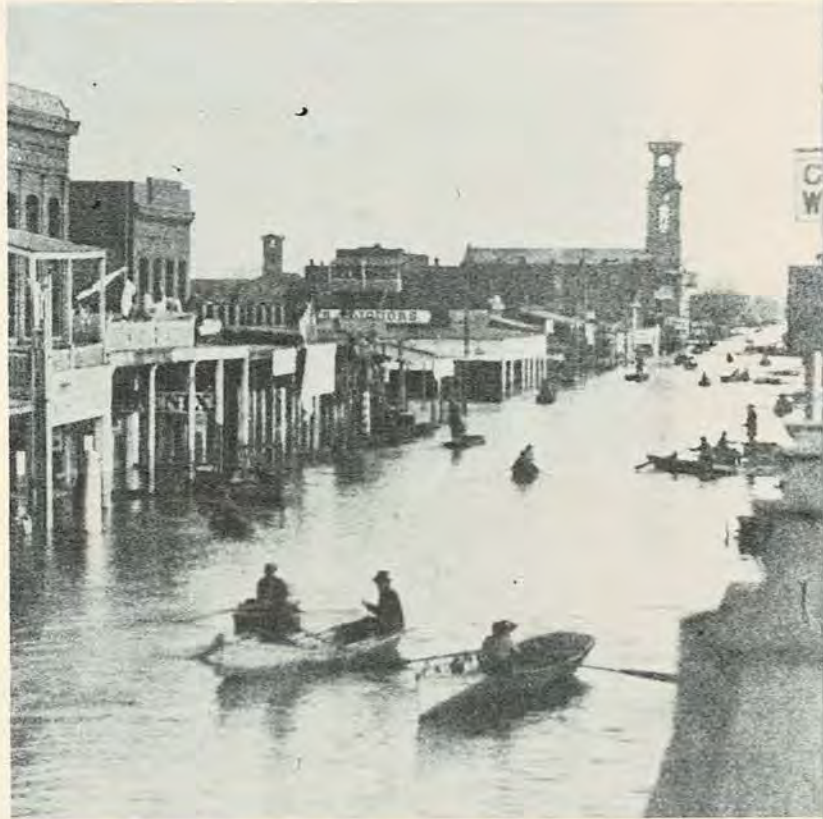
Flooding in the 1850's, dramatized the need for flood control measures.
