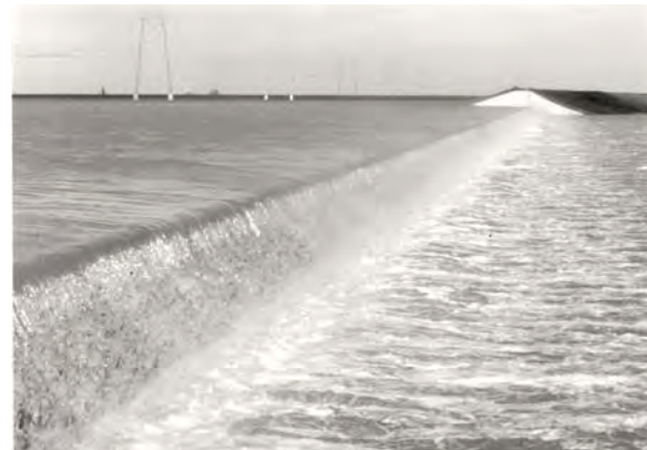
Figure 10, Cache Creek Settling Basin Weir, March 1995
