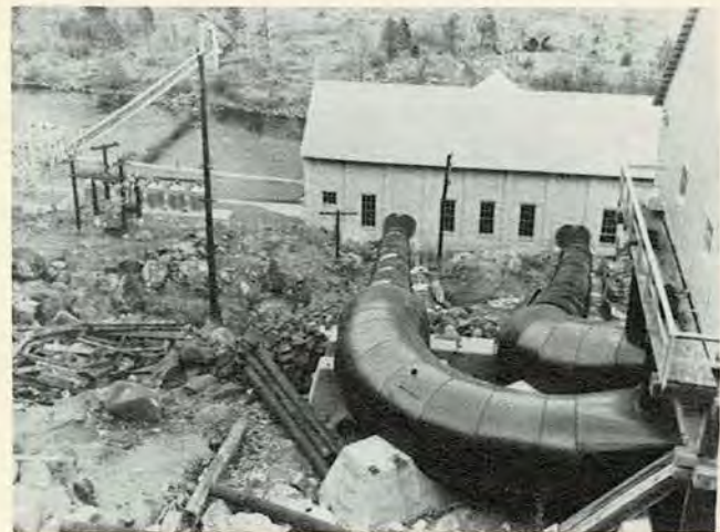
View in 1933, of Farad Powerhouse and penstocks.
