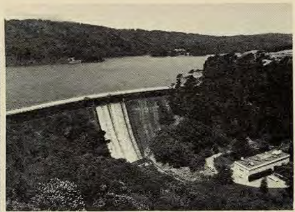
Crystal Springs Dam today. The San Andreas fault runs through the middle of the reservoir behind the dam. Despite an eight-foot shift in 1906, the dam survived undamaged.
