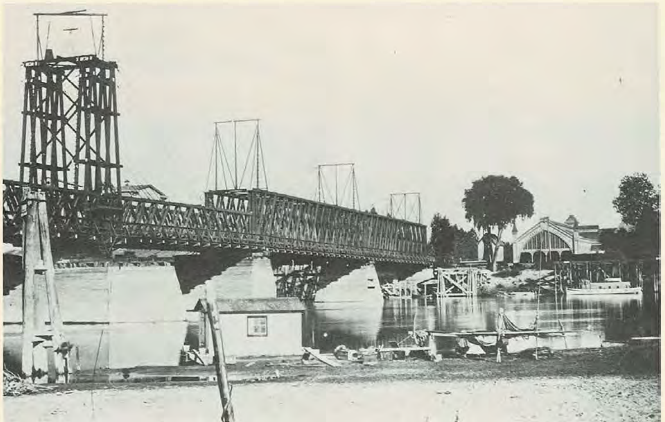
Construction by the Central Pacific of the predecessor to the I Street Bridge.
