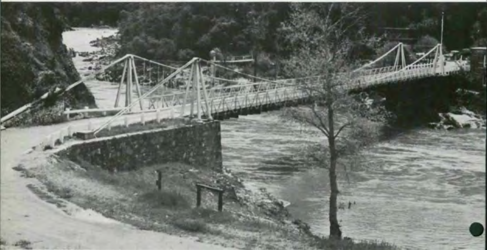
Bridge and toll house before dismantling.
