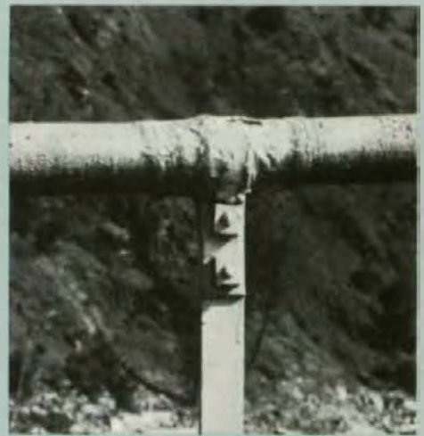
General appearance of cables throughout the bridge.
