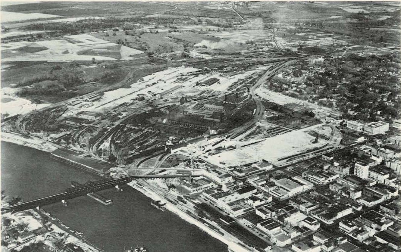
Aerial view of Southern Pacific complex taken in 1925.
