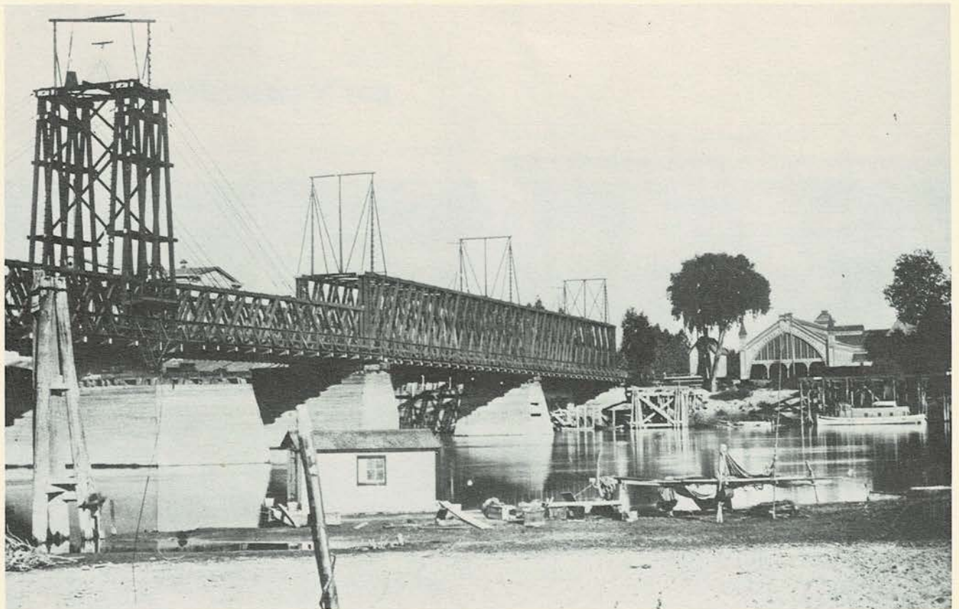
Construction by the Central Pacific of the predecessor to the I Street Bridge.
