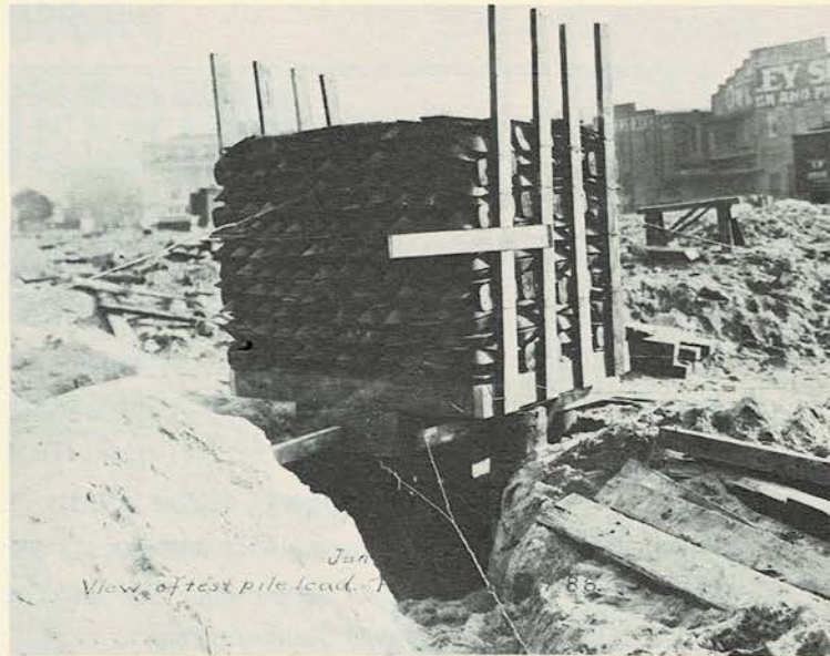
Pile bearing tests in 1925, for the Southern Pacific Depot.
