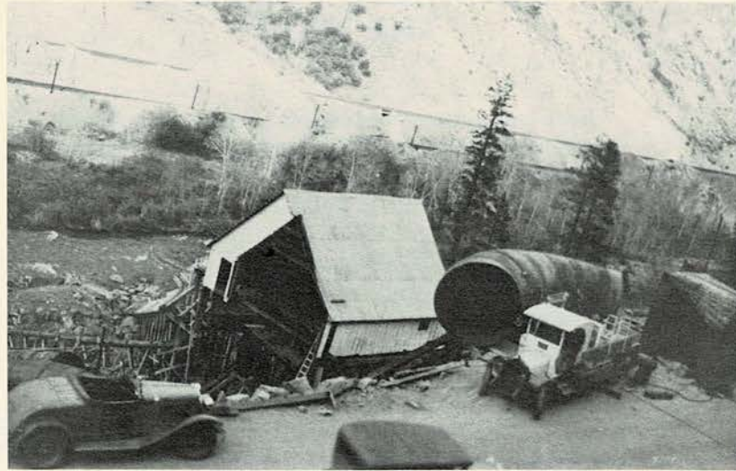
Penstocks ready for placing at the Farad Powerhouse.
