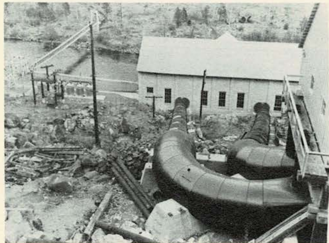
View in 1933, of Farad Powerhouse and penstocks.
