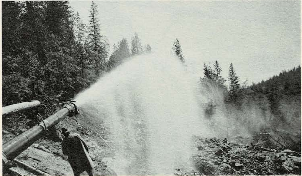
Hydraulic monitor being used to wear down gravel banks.
