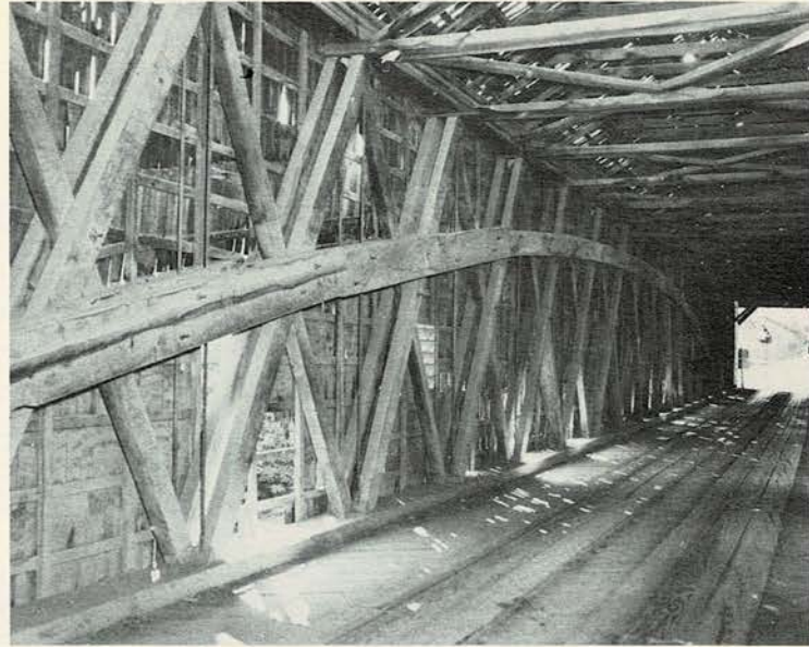
Interior of Bridgeport Bridge showing arch and truss design.
