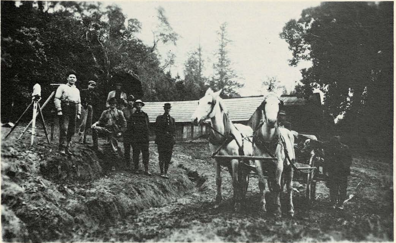
A pioneer surveying and route location crew.
