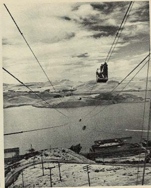
Painting the power cables is a constant task. Work begins from south tower (left) and proceeds northwards across the straits (right).
