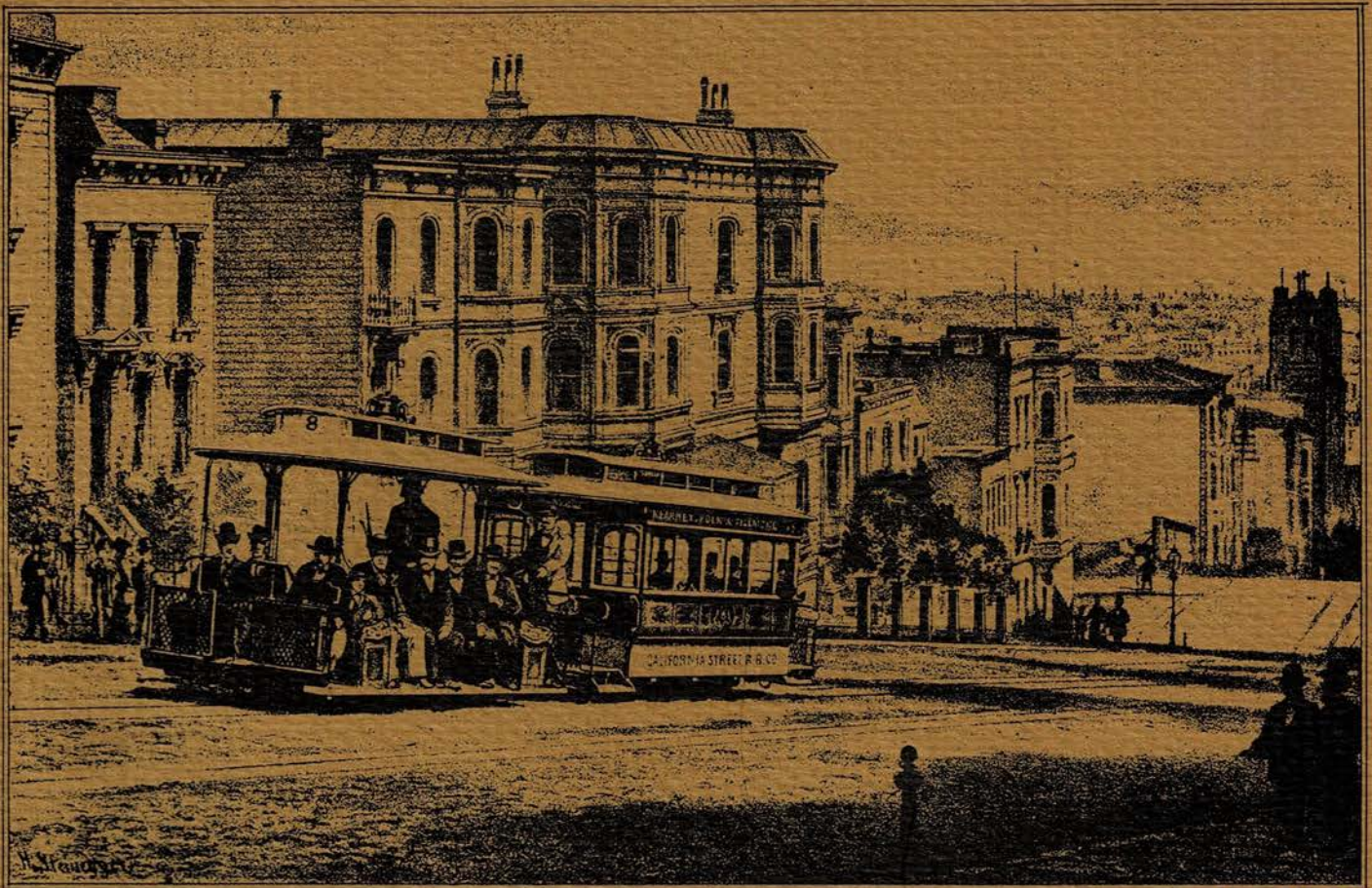
CALIFORNIA STREET WIRE ROPE RAIL ROAD. STEEPEST GRADE 18 FEET IN 100 FEET.
