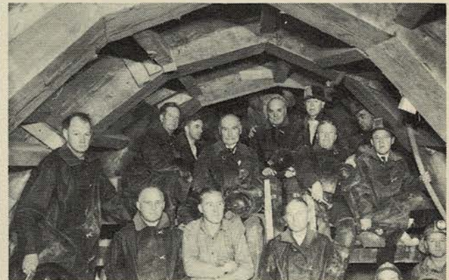
Tiny Niles Dam (top), shown under construction in 1897, is the first point of diversion for Alameda Creek water. (Above) A tired looking Michael O'Shaughnessy (second row, fourth from left) attended the holing through of the Coast Range Tunnel on January 5, 1934.
