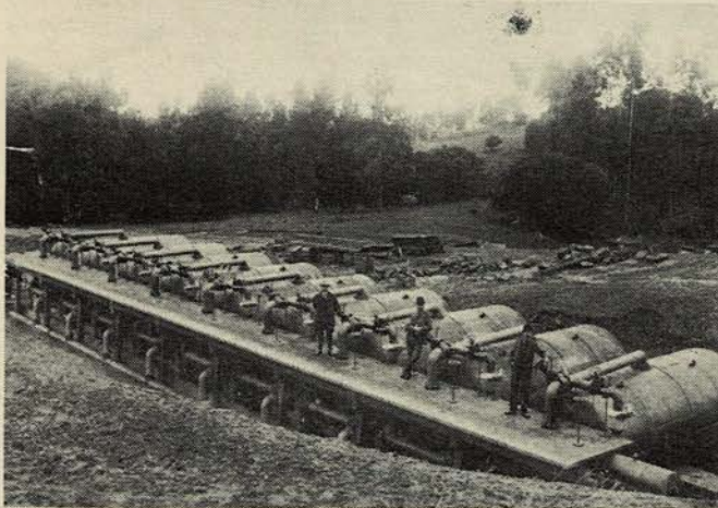
Water from Chabot Dam went through a filtration system, one of the West's first, before going into city mains.
