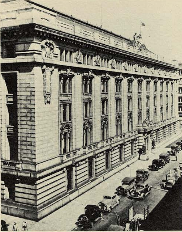
The imposing Italian Renaissance style of the Custom House made it the architectural centerpiece of San Francisco's post-1906 Financial District.
