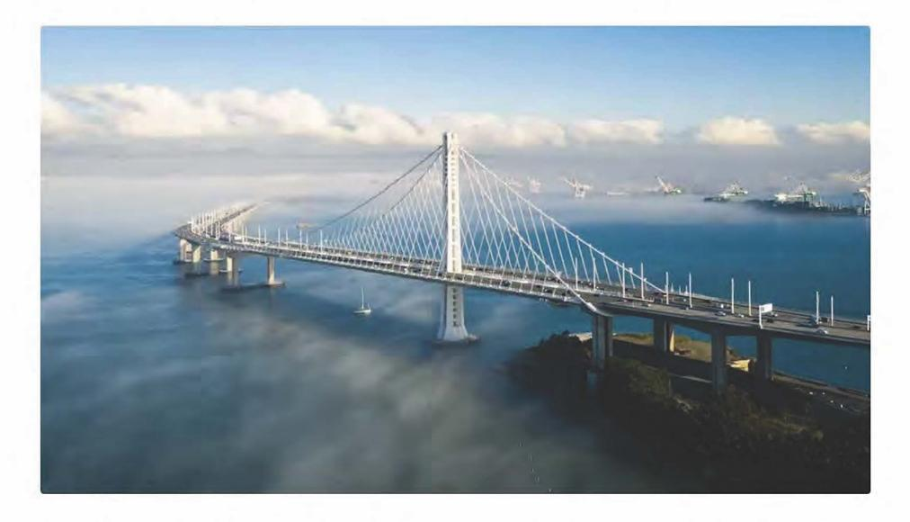
The San Francisco-Oakland Bay Bridge is made up of two bridge segments: a skyway structure/single anchored suspension bridge between Oakland and Yerba Buena Island, and a suspension span from the island to San Francisco. Connecting the two is the largest diameter bore tunnel in the world.
