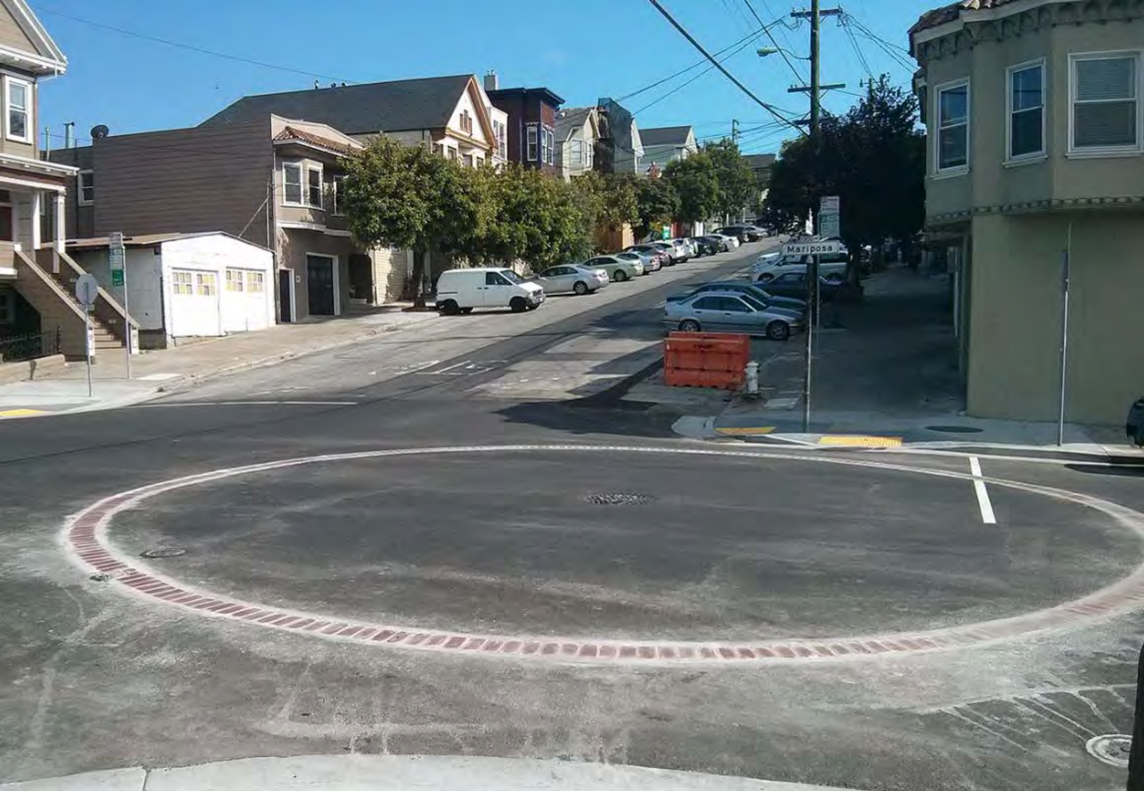
Brick Circle Indicating Underground Cistern
