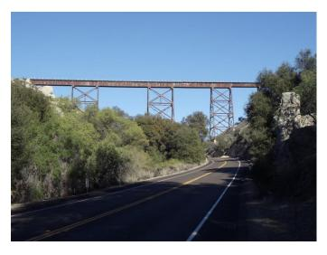
3 and 3-1/2. A massive landslide in March of the same year completely blocked Tunnel 15 in the gorge requiring a permanent bypass of the tunnel and construction of now famous 185 foot high timber pile trestle across Goat Canyon.
