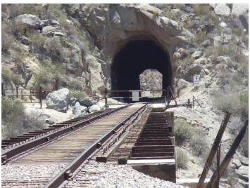
By far the most challenging and expensive section of railroad to construct was in Carriso Gorge. This 11 mile section clinging to the side of the gorge featured 17 tunnels totaling over 2.5 miles, 14 trestles and cost \$4 million alone. The last spike was finally driven on November 15, 1919 and the original construction was completed at a total
