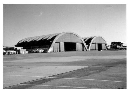
With war clouds looming on the horizon, the U.S. Navy's Bureau of Yards and Docks decided in 1940-41 that a new type of hangar design was needed to protect their aircraft. The main goals were to design a hangar that could be constructed relatively quickly and economically, had a long clear span to accommodate newer larger seaplanes and provided the flexibility to be adapted to
