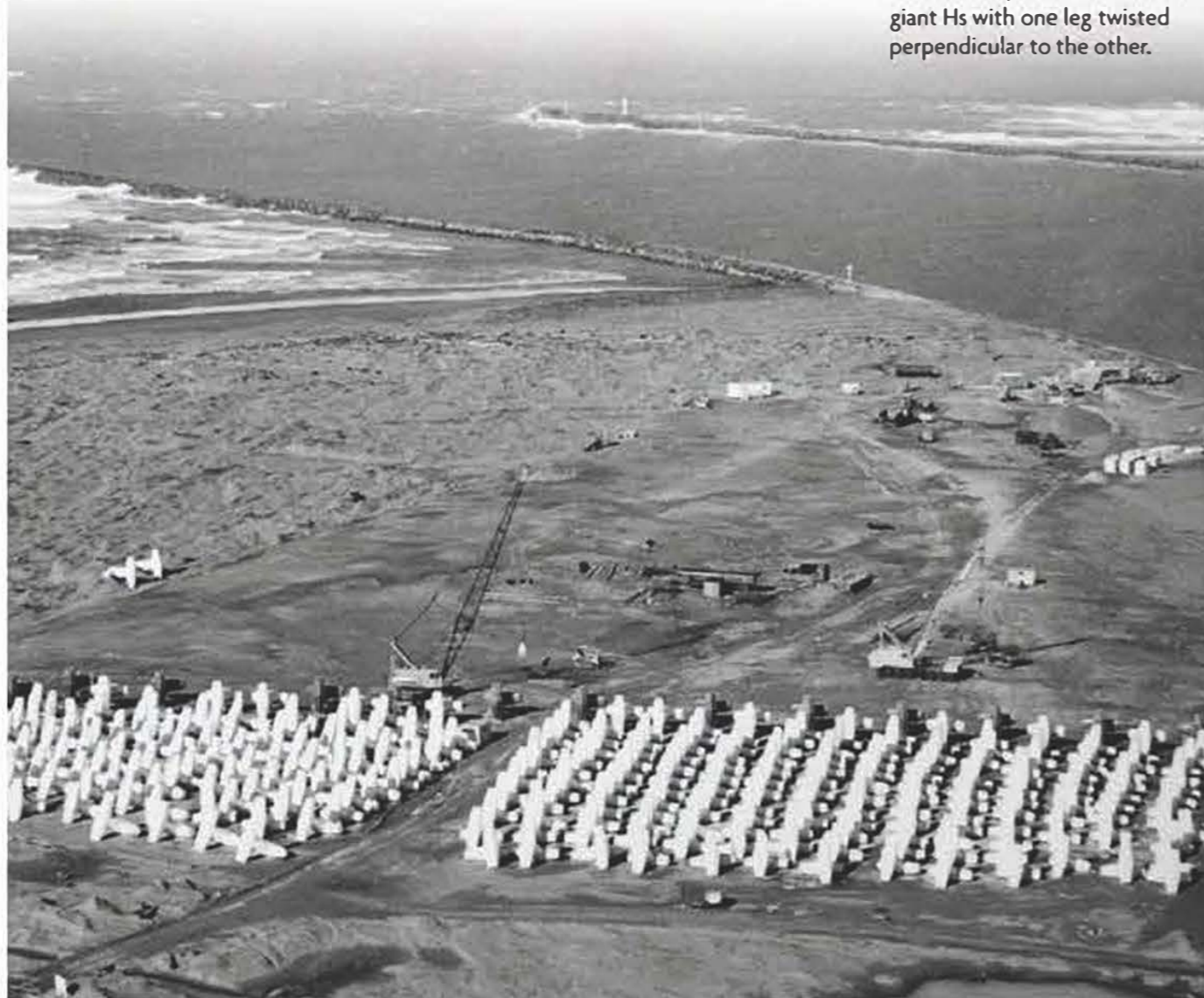
THOUSANDS OF DOLOSSE WERE MADE IN A CASTING YARD ON THE SOUTH SPIT BEFORE BEING TRANSPORTED TO THE SOUTH AND NORTH JETTIES. PHOTO COURTESY OF THE U.S. ARMY CORPS OF ENGINEERS
