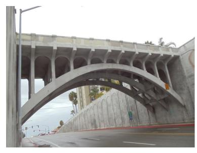
The bridge's most distinguishing design feature is a set of three parabolic reinforced concrete ribbed arches beneath the roadway deck. Hinged at either end and at mid-span and known as the "Thomas Three Hinge Arch" system, the thick concrete arches support a series of columns that are joined at the top by smaller semi-circular spandrel arches. The ribs and arches support the roadway's concrete deck above a
