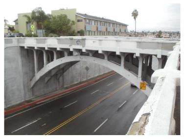
Designed by engineer James R. Comly under the supervision of City Engineer William R. Rumsey, the open-spandrel arched concrete bridge, with its flanking blind-arcade reinforced concrete retaining walls and Mission Revival style graceful three-hinged ribbed arches anchored deep in the opposing embankments, also possesses historical significance for its design and engineering. Although the electric streetcars no longer pass under it, the Georgia Street
