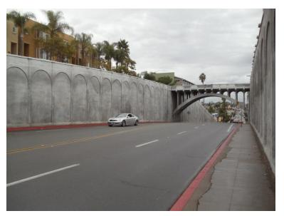
end to 34 feet where it reaches the Georgia Street Bridge. Adding stability is a series of engaged pilasters at 10-foot intervals along the wall's surface.
