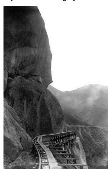
On July 5, 1895 the gate of the reservoir was opened and the new system was in operation. It wasn't long before problems with the somewhat crude system were realized. Water loss from leaky flumes, gopher holes, and percolation resulted in only about 60 percent of the diverted river water reaching the dam. In 1897 the unlined portions of the canal was either lined with cement plaster or replaced with pipe in an effort to improve deliverance. In addition, repairs to leaky flumes were made.
